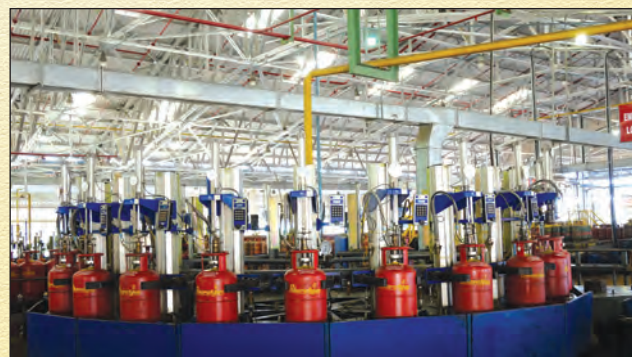
LPG Bottling Plant
