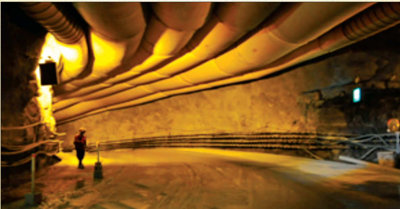
Access tunnel to Strategic Crude Reserve facility at Padur, Karnataka
