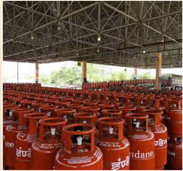
LPG Bottling Plant at Dhanaj
