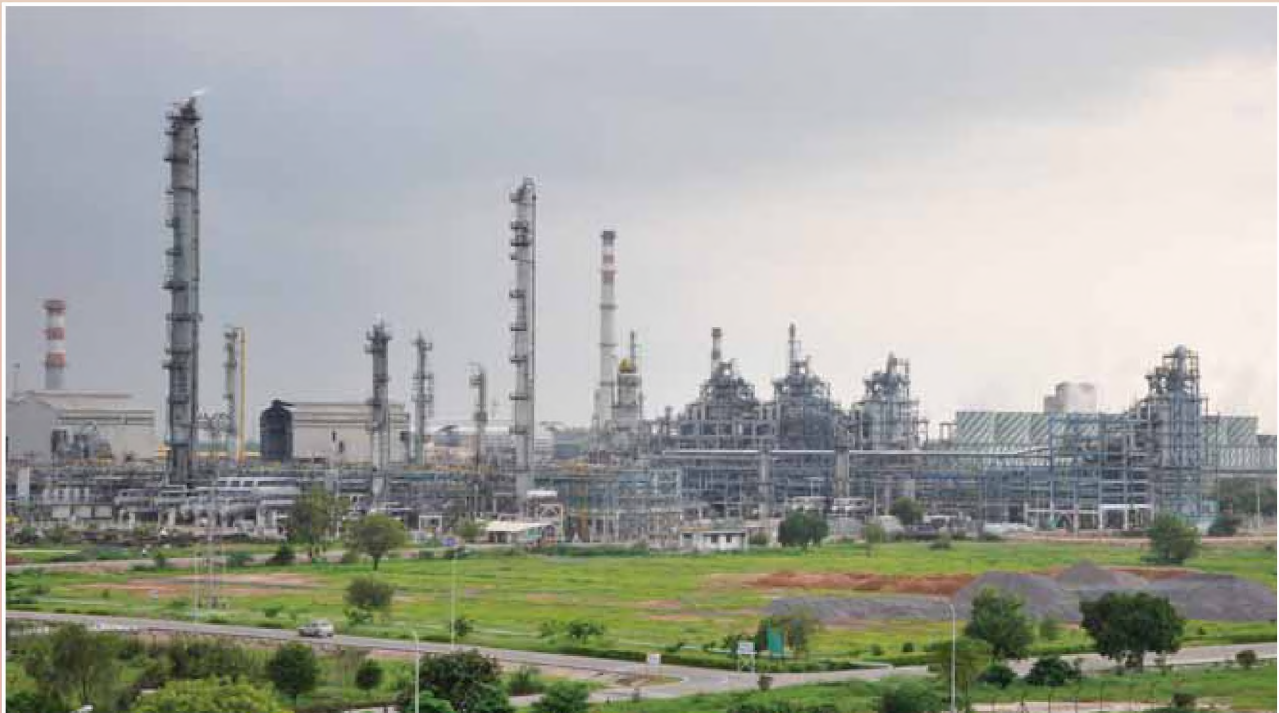
A view of GAIL's Petrochemical Complex at Pata, District Auraiya, Uttar Pradesh
