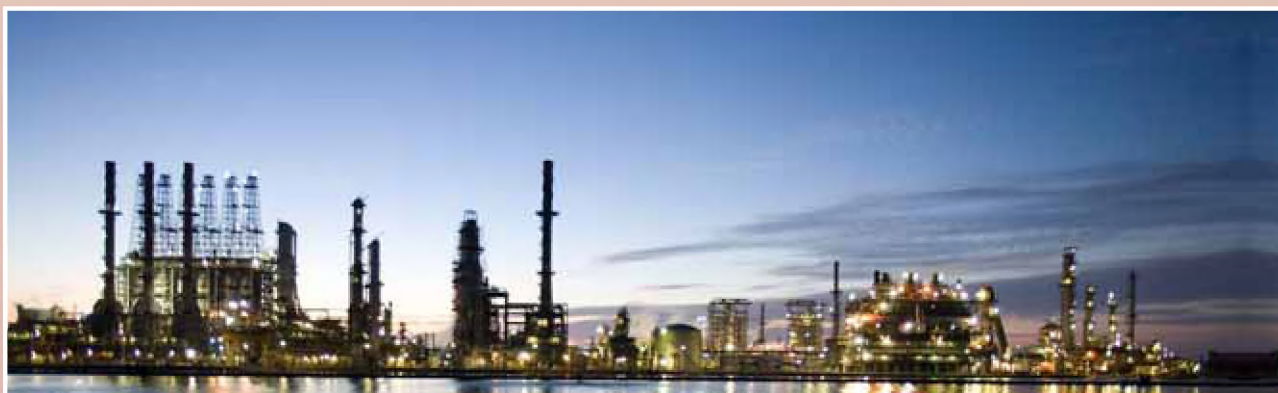
Kochi Refinery of BPCL
