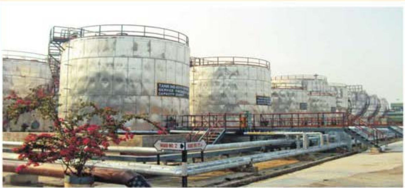
Tank Farm area of Wax Plant, Numaligarh Refinery Limited
