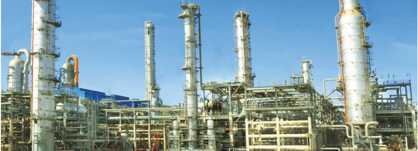
Petrochemical Plant at Dahej Gujarat
