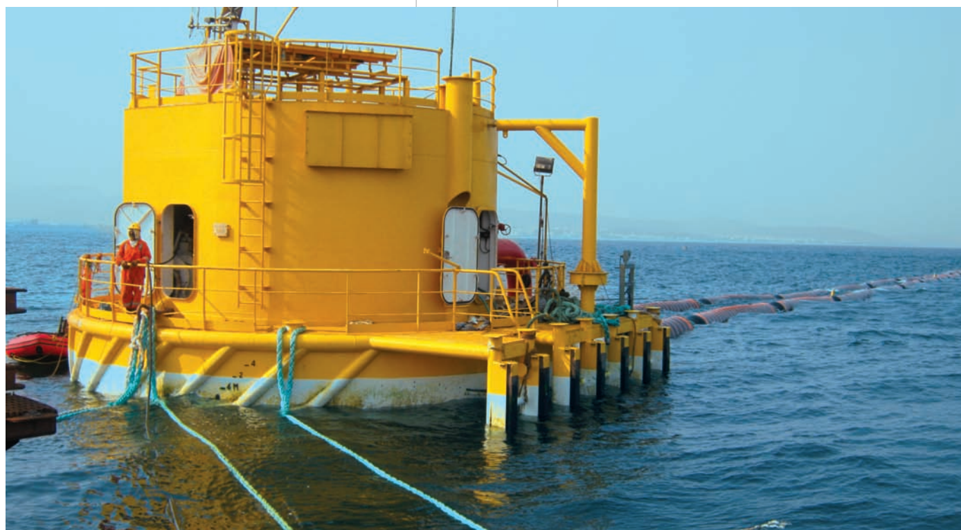
Single Point Mooring at Visakhapatnam
