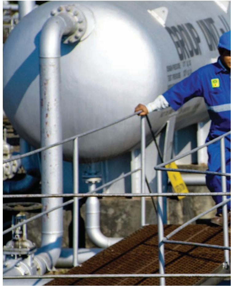
Men at work at an Installation
