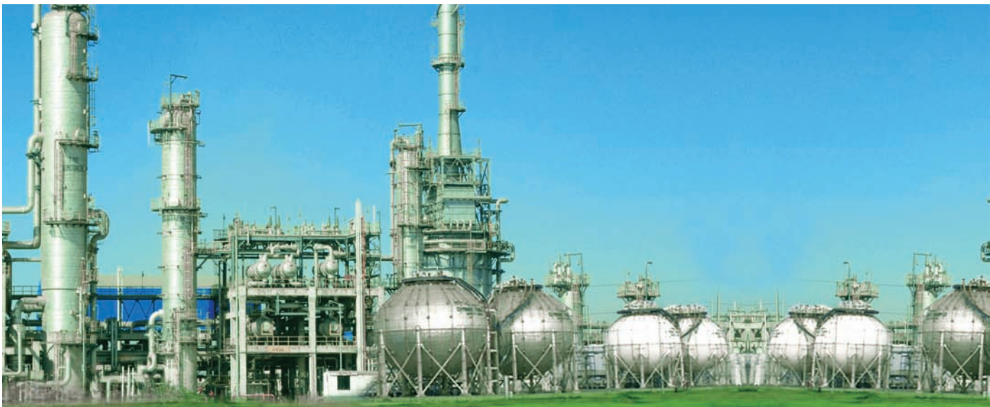
Panoramic view of C2-C3 Extraction Plant at Dahej, Gujarat
