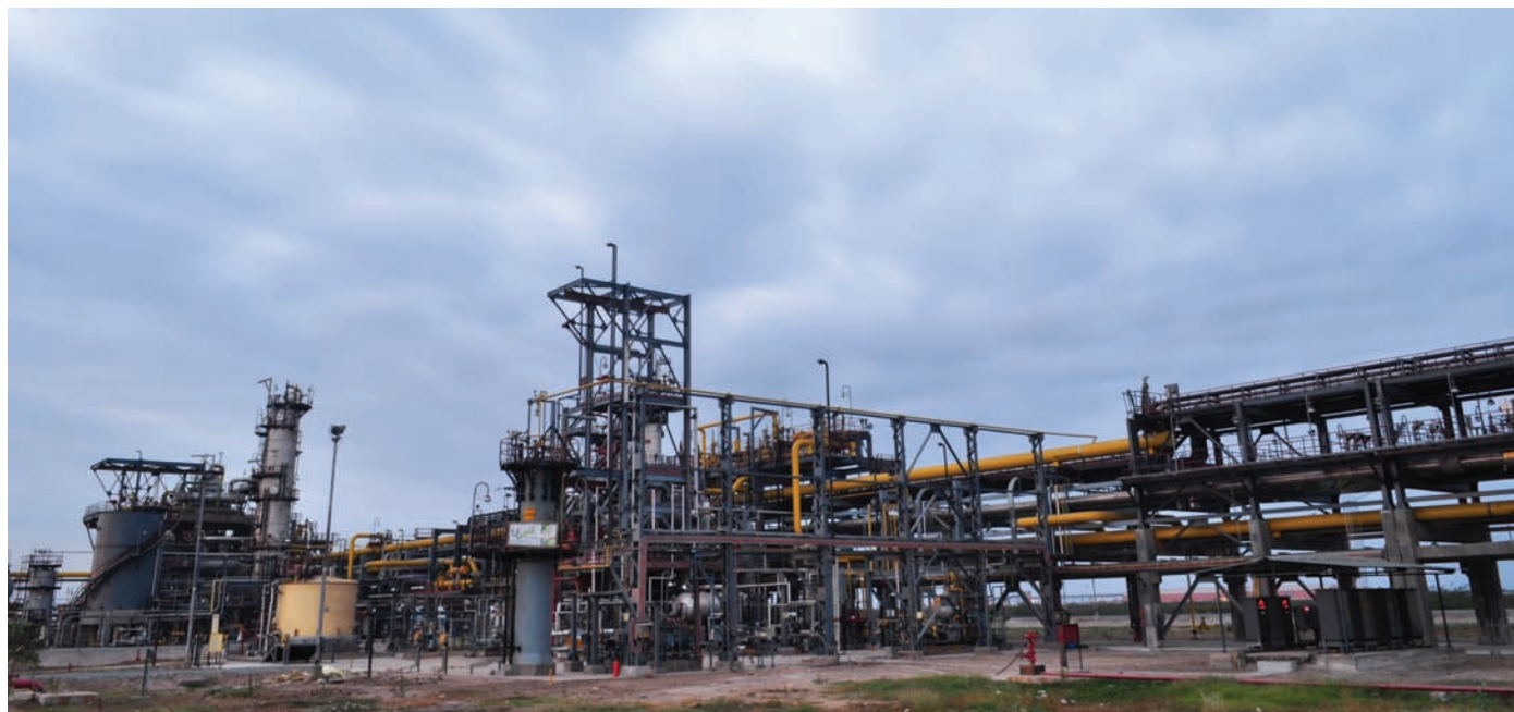
Expansion Project of Gas Process Facility at Hazira, Gujarat
