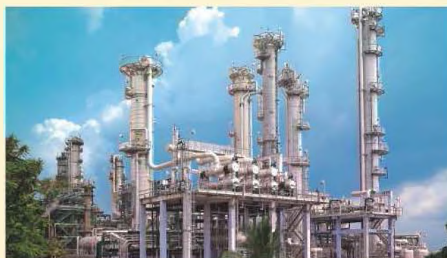
BPCL's Kochi Refinery
