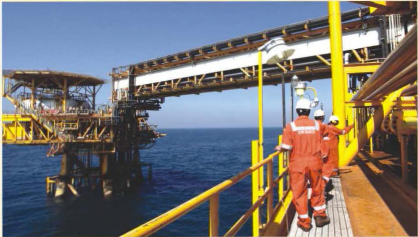
Round the clock vigil on ONGC's Offshore Platform in the Western Offshore
