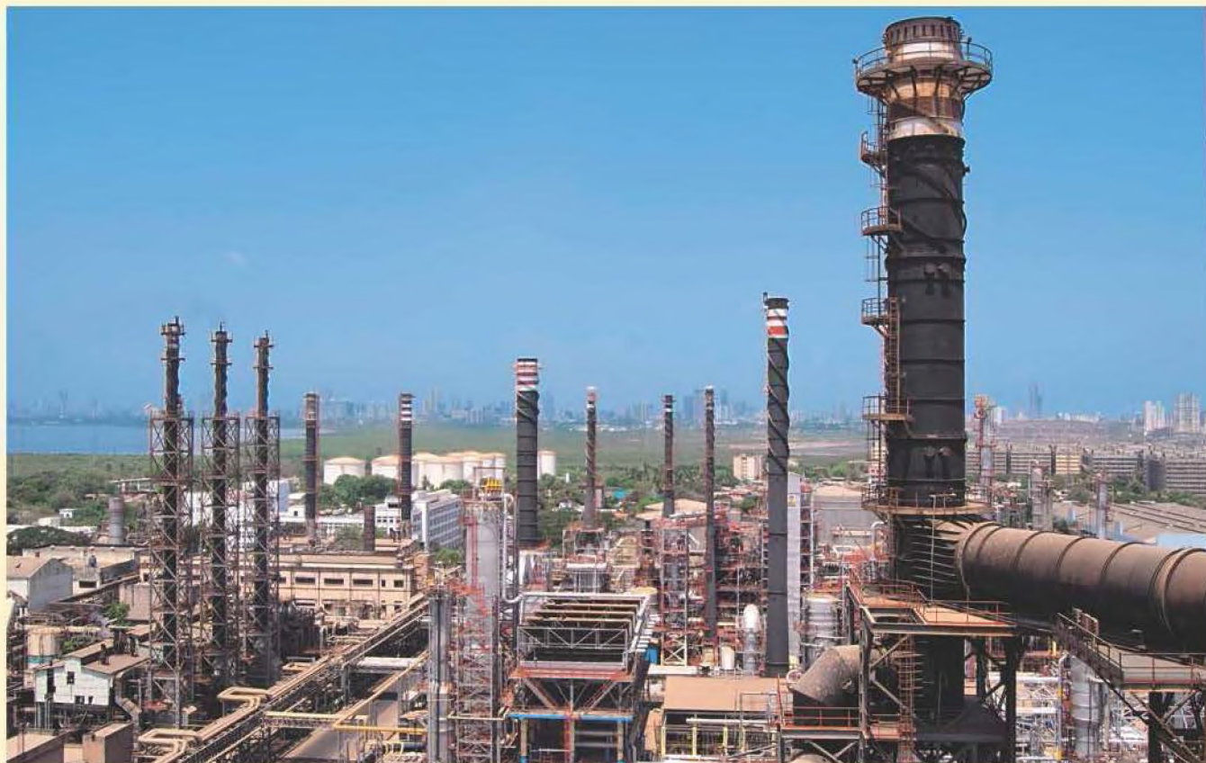
BPCL's Mumbai Refinery
