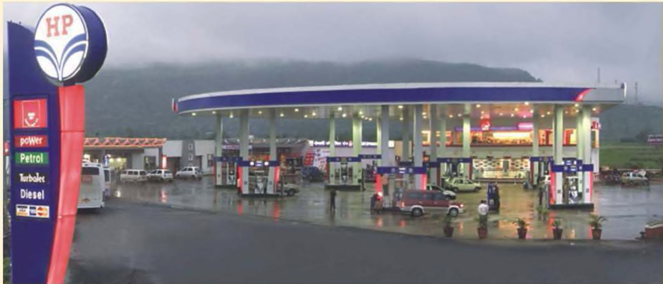
Club HP e-fuel station celebrates a future full of energy
