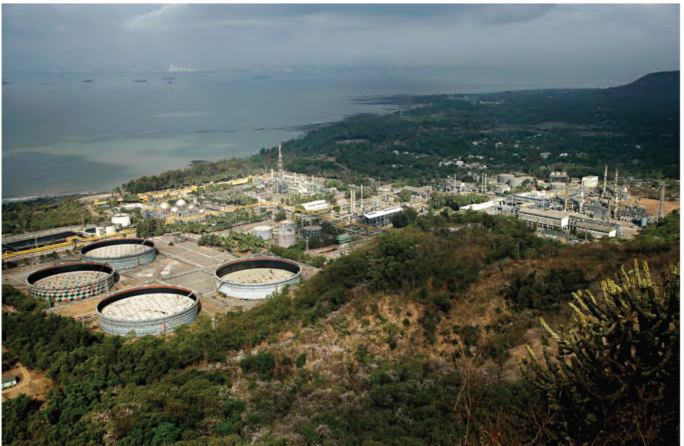
Aerial view of ONGC's URAN Plant
