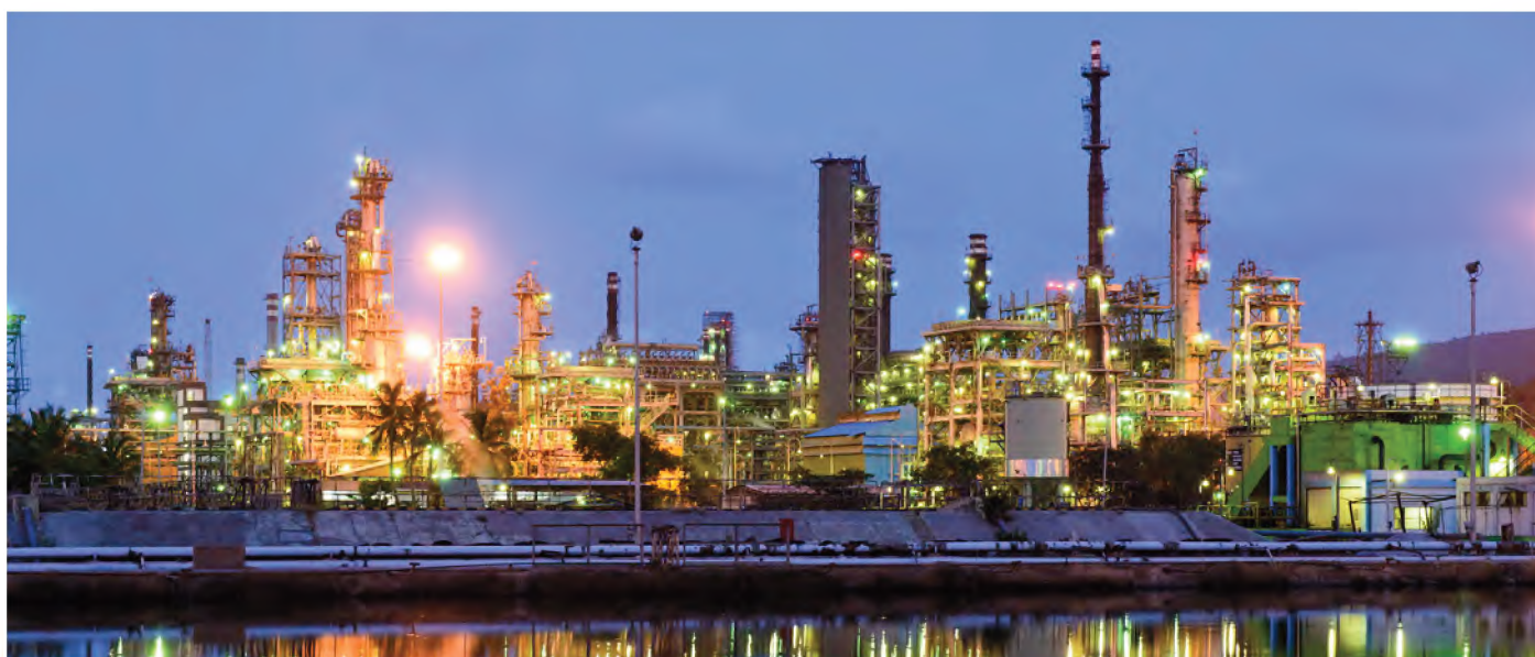
HCL Visakh Refinery
